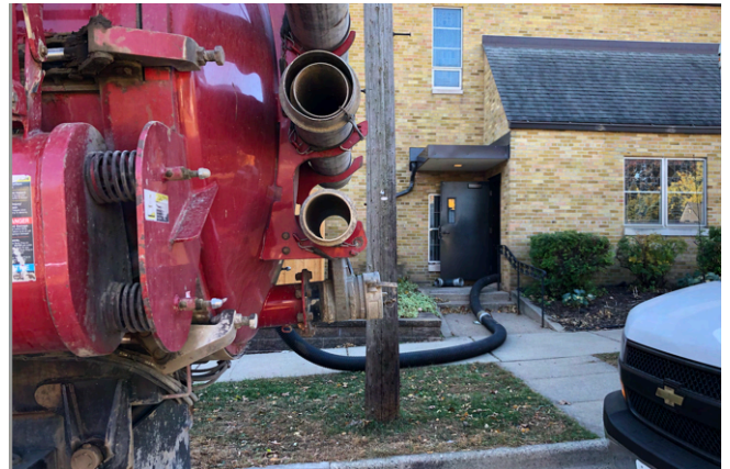
Vacuum pumper “digging” out the elevator pit.
