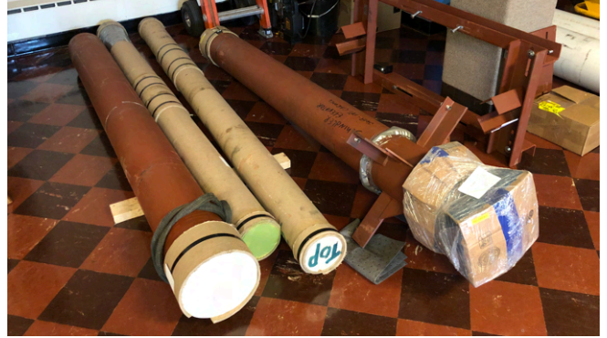
New elevator jack and casing ready for installation
